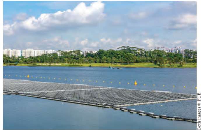
ABOVE: The 1.5-MWp Lower Seletar Reservoir floating solar PV system.
