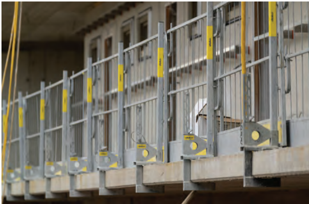
ABOVE: The Edge protection Z provides safety at the edge of a building.
