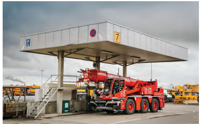
The filling station at the Liebherr plant in Echingen has been converted to HVO fuel.
