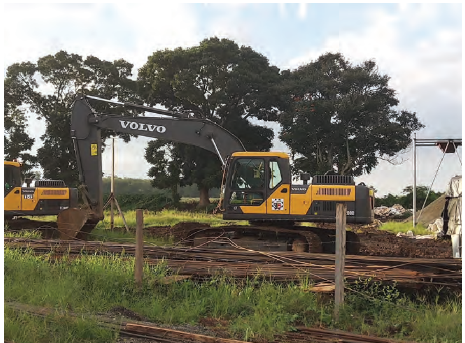
One of RFB Construction Company's Volvo EC200D crawler excavators.
