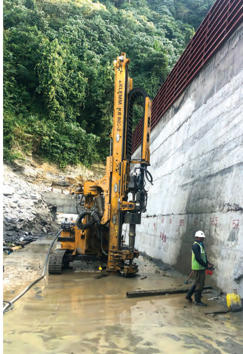
ABOVE: A Klemm KR 909 drill rig being used by Bauer to carry out drilling and injection work on the project.
